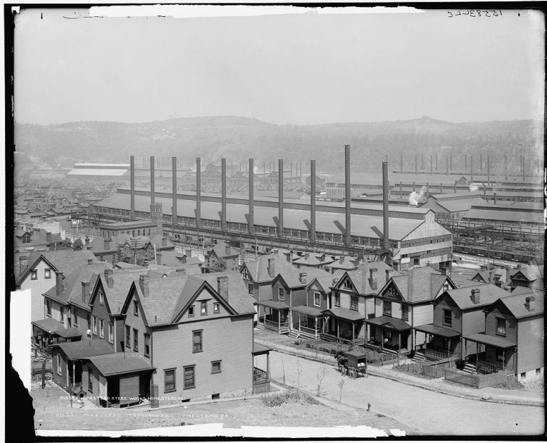
Figure 3: Photo of Homestead Steel Works (1900-1910)
